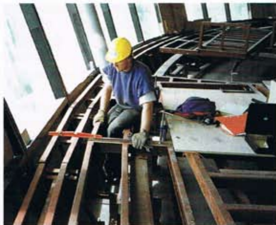
Above right and facing page: The revolving restaurant runs on a highly-advanced rotating floor system designed and installed by Wilson Engineering. It was completely pre-assembled off site to ensure the accuracy of the components. Dominion Constructors built the fire-resistant floorboards for the rotating floor. The carpet and upholstered upstands were installed by Hills Floorings.
