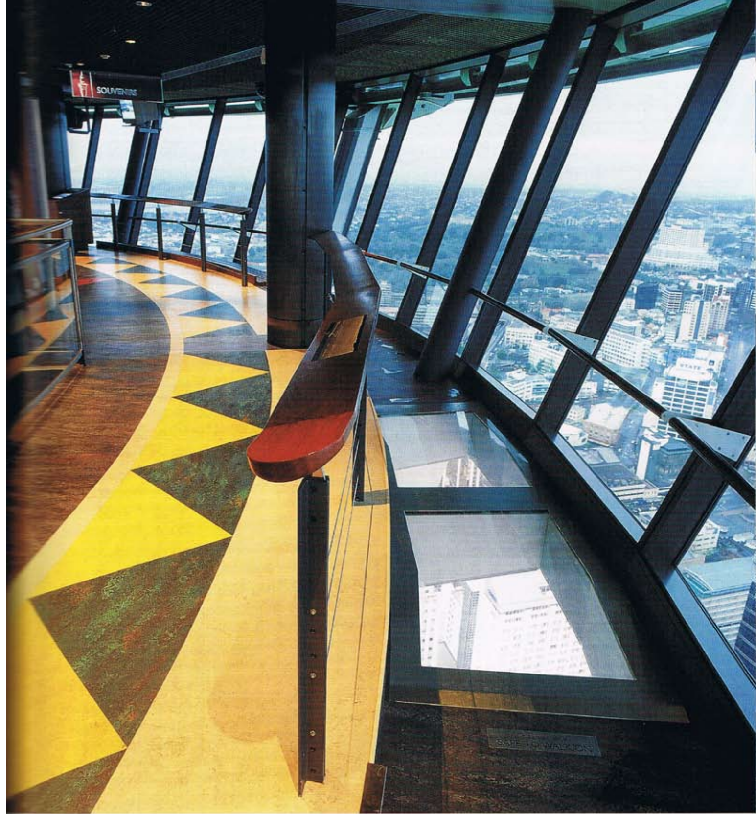
Above: G James installed four glass viewing ports at each compass point in the floor of the main observation deck. The 44mm-thick starphire glass is specially made to handle heavy foot traffic.
