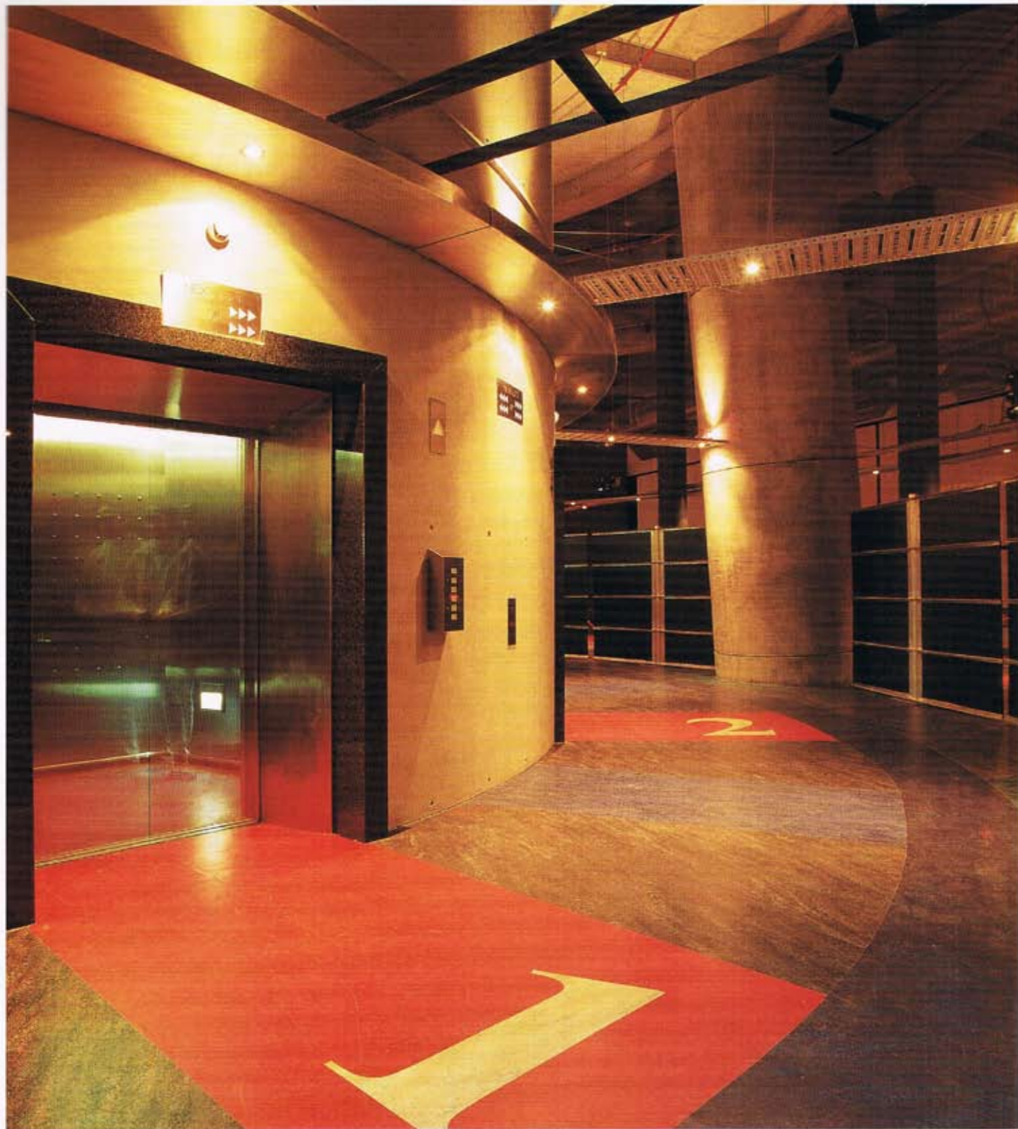
Above: The bold marmoleum floor design, installed by Hills Floorings, helps to indicate the three passenger tower lifts.
